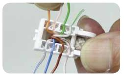
3. Separate the wires and secure them to the adapter body according to the wiring standard you are implementing.
