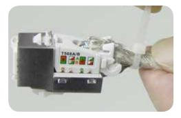
8. Secure the field cable to the adapter strain relief tab using the zip ties provided. Cut off excess cable tie material after securing the wire.
