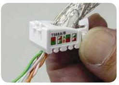
2. Insert the stripped back wire through the adapter body assembly.
