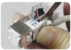
7. Cut off any excess wire from the edge of the closed adapter assembly.
